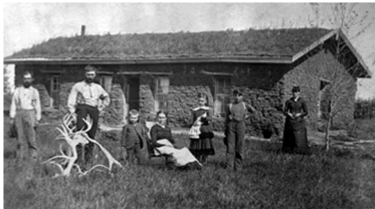
A family poses before their sod house in Nebraska in 1887. Made from strips of earth and plant roots collected with a plow, sod was plastered with clay and ashes in a brick-like pattern. Sod houses were common in the Western U.S. plains because timber was scarce.
